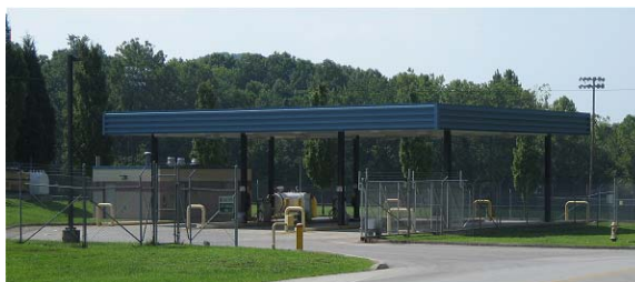
Top: A sticker that the city has developed to show their use of biodiesel. Bottom: The refueling facility off Blank Drive.
