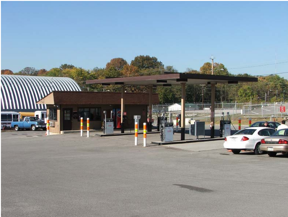
Picture 1. The main refueling facility for the county where a bio-blend is provided.
